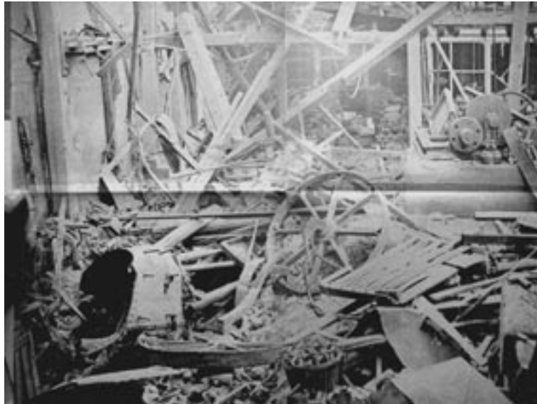
Figure 3: The exploded boiler. (Boiler explosion, Paris, 1858, Archives nationales).
